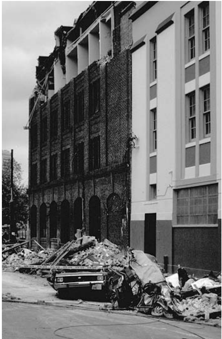
Cars crushed by collapsing brick facade near Fifth and Townsend Streets after the 1989 Loma Prieta earthquake. At this locality, five people were killed while leaving from work.
