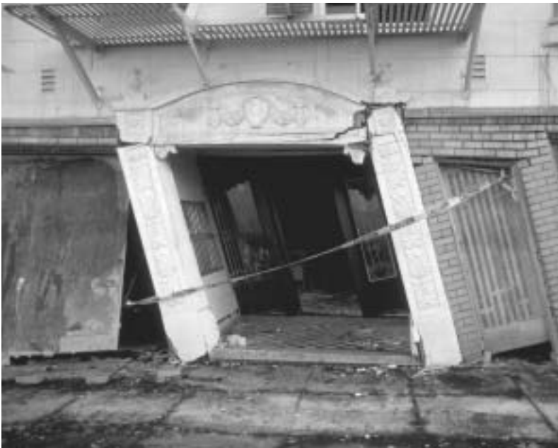
Entrance and garage level of a Beach Street apartment complex in danger of collapse after the 1989 Loma Prieta earthquake, Marina District.
