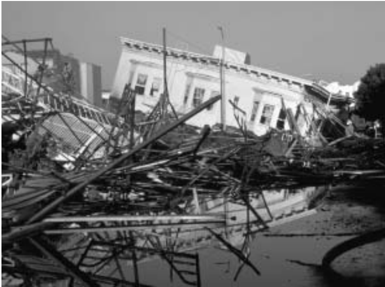
Ground view of a collapsed building and a burned area after the 1989 Loma Prieta earthquake, Beach and Divisadero Streets, Marina District.
